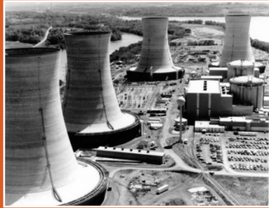
The Three Mile Island Power Plant in Pennsylvania, which in 1979 was site of the worst nuclear power plant incident in US history.
